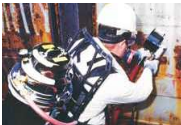
Air Backpack model with RotoPeen tool removing rust from a steel structure.
