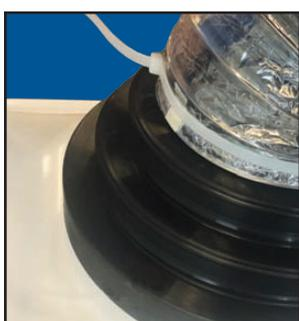
Place flexible duct onto reducer and secure with duct strap
