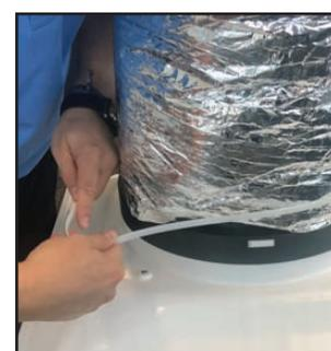
Use second duct strap to secure insulation
