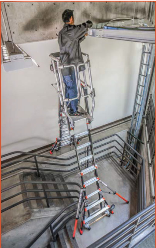
Stair access made safe
