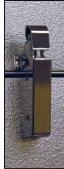
Spring actuated door closer
