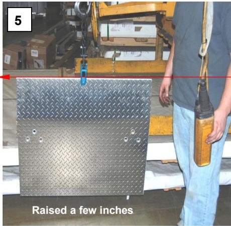
This side of the sheet material hangs lower than the other. Return the material to the ground (or other supporting surface) and reposition the clamp by moving it closer to this end.
