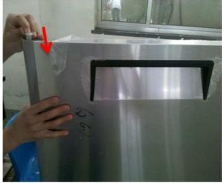
1∠.Aπer installing the door,screw the top hinge(follow the arrow.)
