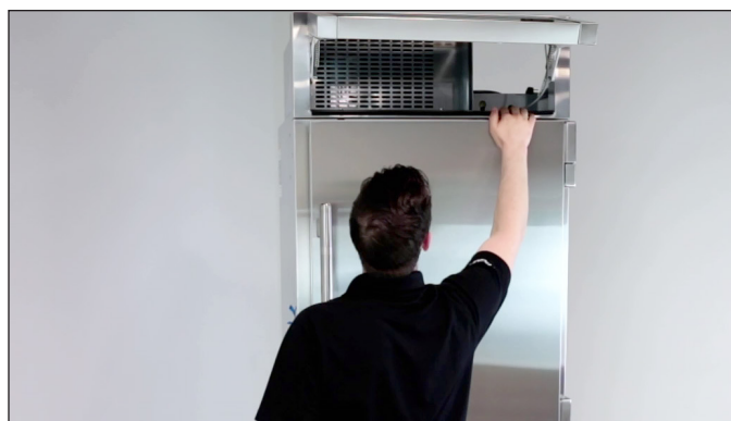
FIG. 3. Be sure to inspect behind the rainshield.
