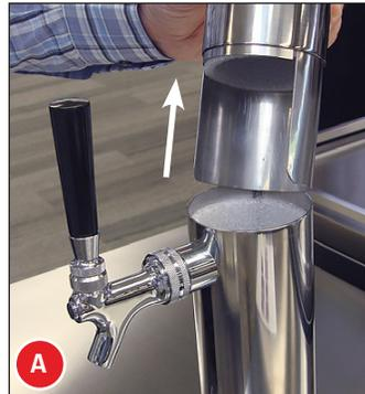
**Fig. 7.** Route the air hose through the draft tower from below.
