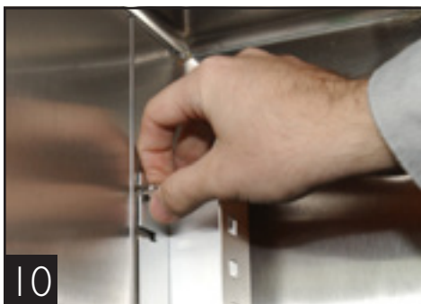
Pilaster installation (side wall of cabinet)
