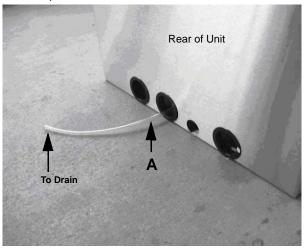
4. Verify the tubing is not kinked and then secure tubing to maintain a minimum 1" (2.5 cm) air gap at the drain. Follow any applicable local or national codes.
