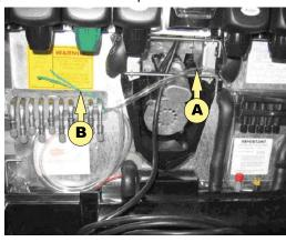
3. Depending on drain location route the tubing through the tubing bundle cutout or out the back of the dispenser.
