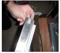
16) Install the door back onto the top hinge and align the bottom of the door with the bottom hinge. Reinsert the bolts into the bottom hinge and secure
