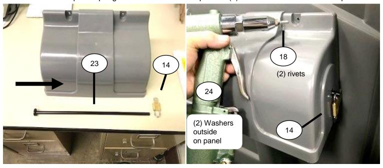
Drill out in center of bottom tabs in PaperGuard hood through panel using #10 Drill Bit. Fasten urinal to panel, use (2) Rivets #11030 inside through holes drilled in urinal / panel & (2) washers #11315 outside on panel.
