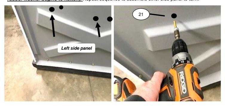
Locate 2 dimples in lower rear section of rear panel. Install (2) Screws #13860 through dimples into tank using of 3/8" Nut Driver bit.
