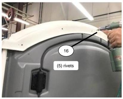
Drill through 5 holes in roof (5 dimples if roof has no holes & panel has no holes) through rear panel using #10 Drill Bit. Fasten roof to rear panel using (5) Rivets #11030 outside on roof & (5) Washers #11315 inside on panel.
