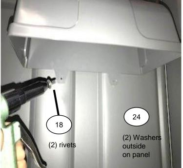
**Step 9: Assemble Roof to panels & front:** Place roof on panels & front as shown. Push roof towards back of cabana so it is tight against front door frame. Drill through 5 holes in roof (5 dimples if roof has no holes) through front *(only through first wall of door frame)* using #10 Drill Bit. Fasten roof to front, use (5) Rivets #22199.T-11 roof shown, T-22 roof is installed the same way.
