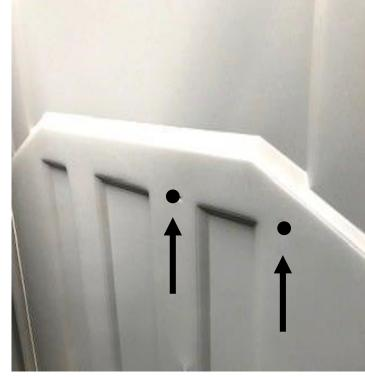
**Step 8: Assemble Paperguard hood to panel (continued):** Install toilet paper rod #1051-699 in Paper guard hood from left to right end with hole in first. Place Padlock #1038-699 on end hole (out from right side of Paper guard hood). Fasten Paper guard hood to panel, use (2) Rivets #11030 inside through holes drilled in top of Paper guard hood into holes in panel & (2) Washers #11315 outside on panel.
