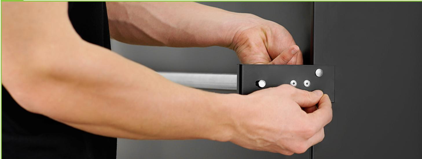
**B** Secure the garment rod with hex head bolt.
