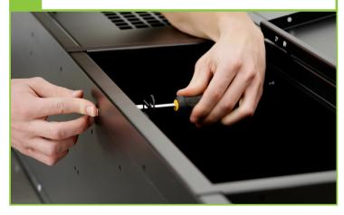
Inside of shelving will need to be bolted to the locker door frame.
