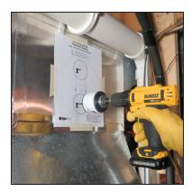
5. Take care to prevent the metal disc from falling into the HVAC system. **NOTE:** If the disc falls into the HVAC system it will not negatively affect its operation.
