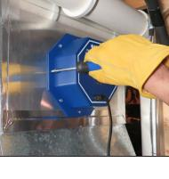
13. Turn the system on (solid line on the switch pressed down) and verify that the LED indicator light(s) are illuminated.
