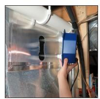
9. Attach the system to duct work with the 8 sheet metal screws using a 1/4" nut driver. Make sure to tighten screws evenly. **CAUTION:** DO NOT OVERTIGHTEN SCREWS.
