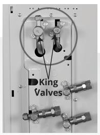
5. Using soapy water (in a spray bottle or with a brush), or leak detection spray, apply to the Quick Connect® fittings at the indoor air handlers and outdoor condenser to check for leaks. If you see bubbles begin to form, this indicates there is a leak. If so, re-tighten the connection accordingly until the bubbles are gone. Please refer to the manual for more detailed information on checking for leaks.
