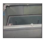
Attach the extension by aligning its edges with the top rail of the interceptor (make sure that all extension edges are sitting onto foam gasket).
