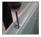
STEP 3: Remove the lid and make a couple of holes in the middle of the long rails of the top interceptor (close to the center pins).
