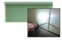
STEP 2: Cut extension to meet required length. Connect the 2 extension halves by using the self tapping screws. (To avoid injury during inside cleaning, tap the screws from inside out).
