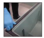
**STEP 4:** Attach the self-adhesive foam gasket on all sides of the top rail of the interceptor.
