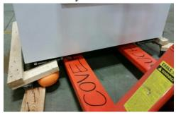
5. Use lifting device to lift the unit high enough to remove pallet and the orange pallet cushions from the back.
