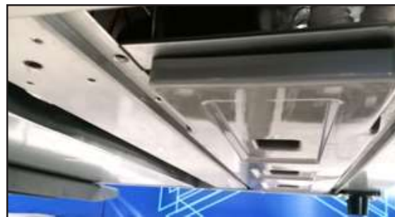
Condensate Pan Installed
