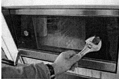
Fig. 3 Loosen the screws to substitute glass
