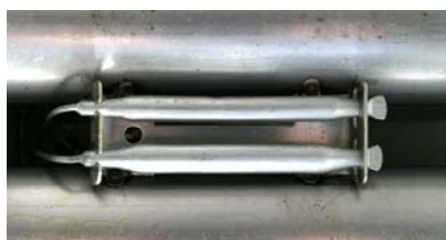
Typical high-limit/sensor probe locations and mounting hardware.
