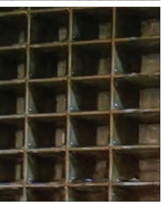
Grid is difficult to clean. A dirty evaporator can cause diminished production, increased service cost and premature equipment failure.
