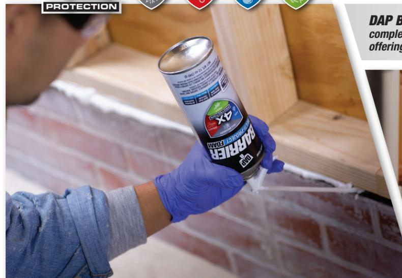
DAP BARRIER™ Spray Foam is proven to offer complete 4X PROTECTION for homes while offering more projects per can and less waste
