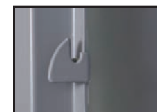
Main door latch hooks welded to frame
