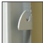
Latch hook is welded to frame
