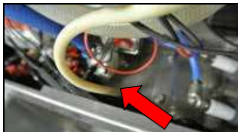
Installed grommet in the hole.
