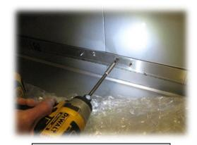
Install the "Bottom Rear Bracket" using the bottom holes for the center pilasters (Above). Install the supplied ¾" long screws into the bottom holes of the Side Brackets to hold the ends of the Bottom Bracket. (Do not tighten these screws at this time. These screws will be tightened after the Back Spacer is installed.)
