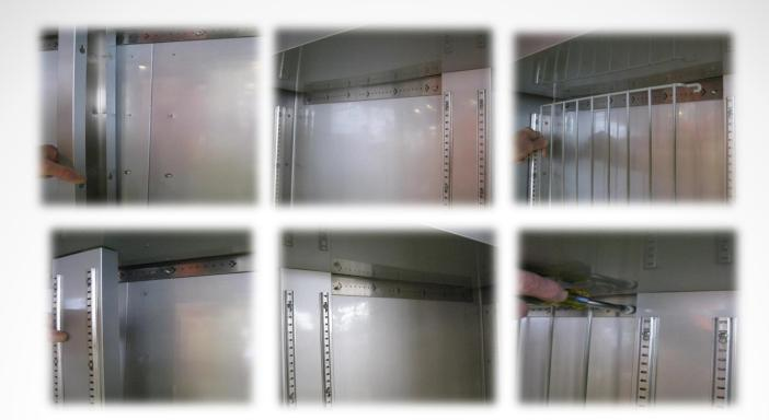
**H2 & H3 Only** - After the top and bottom brackets are installed, the "Rear Pilaster Support Bracket(s)" can be installed.
