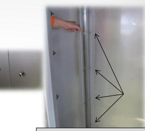
Install (8) of the screws removed in the last step in the 3rd, 5th, 7th & 9th set of holes in the back liner. (Counting down from the top.) The screw head should be 1/8" form the back wall to allow the Rear Pilaster Support to be slid over the keyhole slot.
