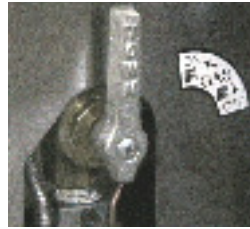
figure B BURNER VALVE IN ON POSITION— ROTATE COUNTER CLOCKWISE TO TURN OFF
