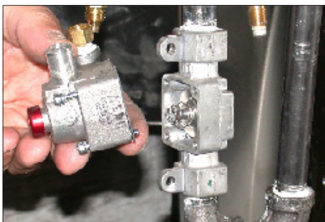
4) Remove the safety head
