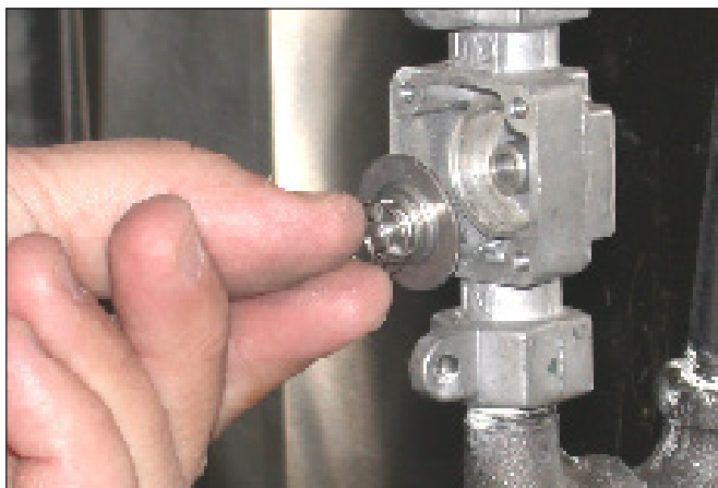
6) Remove and replace the spring/magnet assembly
