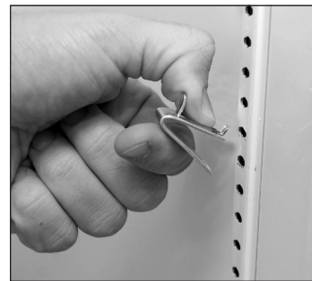
Fig. 1. Installing top tab of shelf clip.
