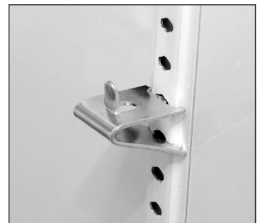
Fig. 4. Installed shelf clip.
