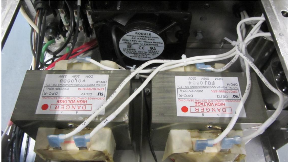
HIGH VOLTAGE TRANSFORMERS – COOLING FAN
