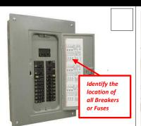
**1.** From your **Electrical Circuit Box**, check and identify the position of all the External circuit breakers or fuses for the oven
