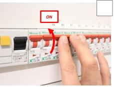
**2.** If you have External Circuit Breakers. Check that all the breakers are in **ON** position. **IMPORTANT!** Call an electrician if the Breaker trip again
