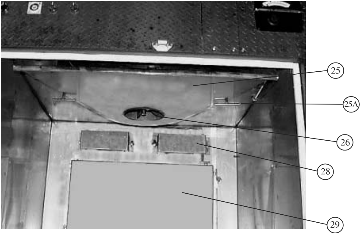
INTERIOR VIEW WITH ALL BAFFLES IN PLACE
