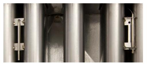
Typical sensor probe/high-limit locations and mounting hardware.
